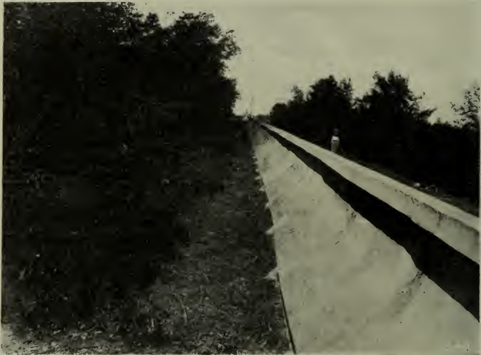
Fig. 9. Sea Wall, Moss Rapid (Looking East). COAST PRESERVATION IN BRITISH GUIANA.
